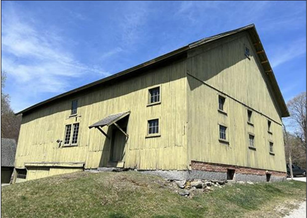
The Green Barn is an English bank barn with an attached wagon shed. The foundation consists of load-bearing Masonry and the framing is hand-hewn post and beam. Materials include brick, cut stone, vertical siding, and asphalt shingles. Historically, the barn was used for dairy agriculture and was built before 1859.
